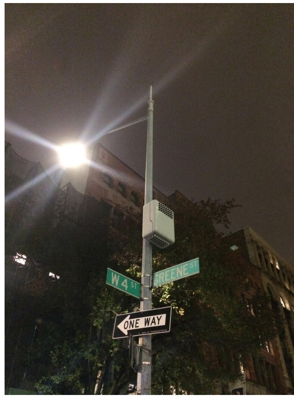
Distributed Antenna System (DAS) Network Amplifier
