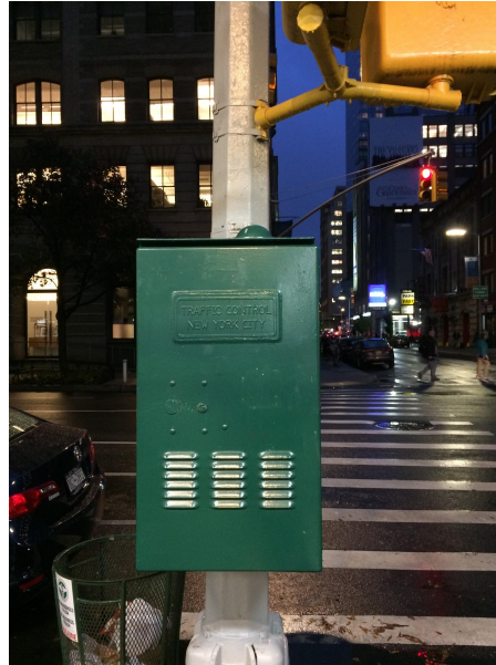
Traffic Signal Controllers (Connected to NYCWIN)
